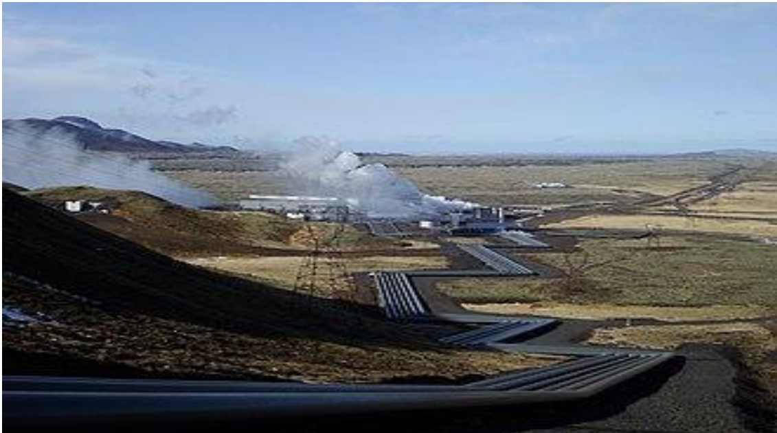
Figure 4 - Hellisheiði Power Station
