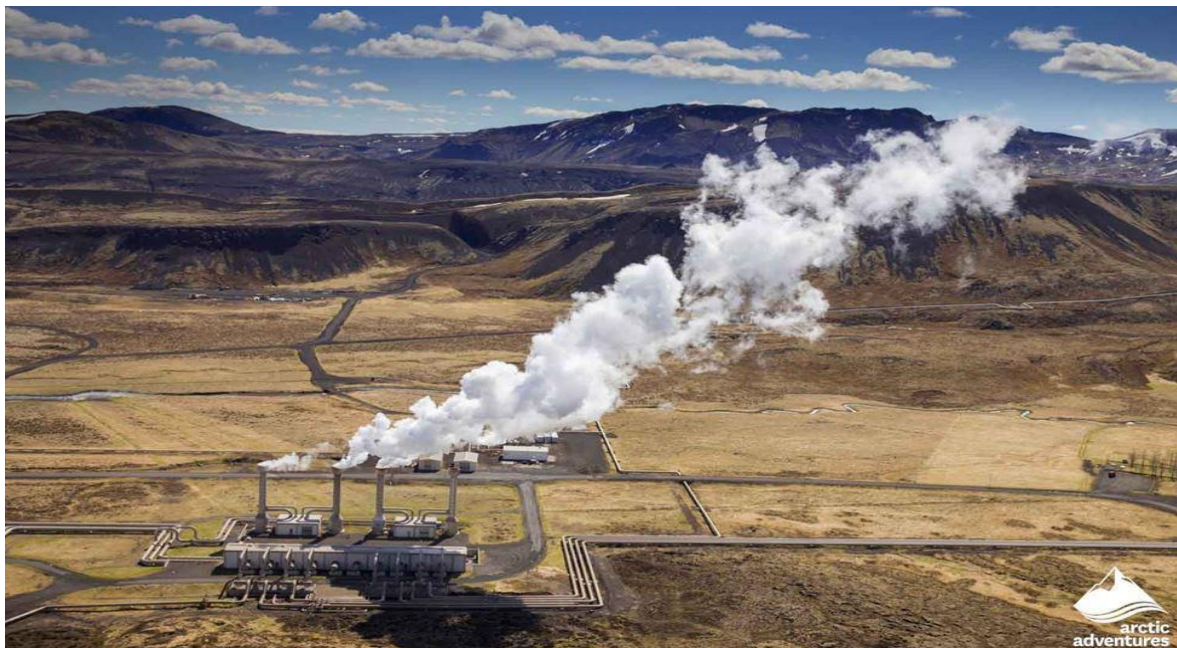
Figure 6 – Nesjavellir Geothermal Power Plant
