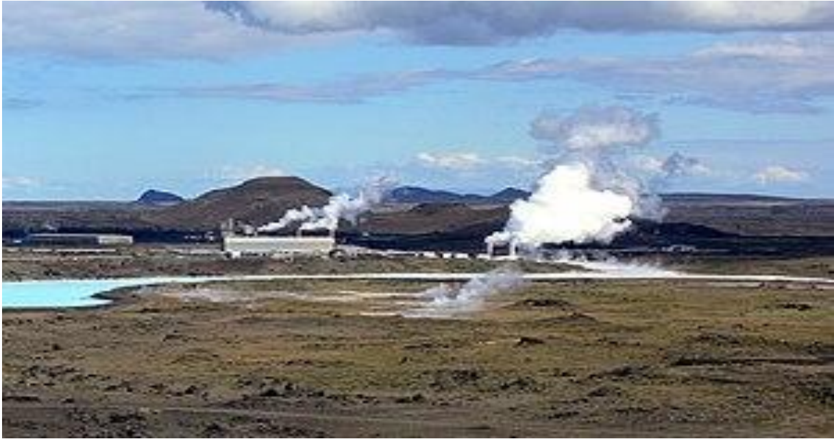
Figure 5 - Reykjanes Power Station
